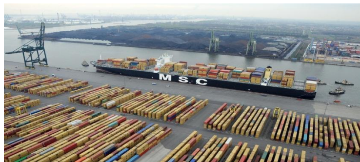
MSC Home Terminal in Antwerp, Belgium
